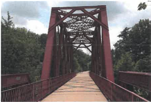
A bridge along Indiana's Monon Trail | Photo by Robert Annis
